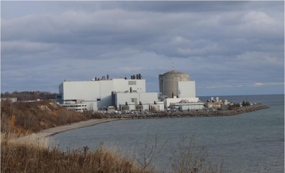
Darlington Nuclear Generating Station, Ontario, completed in 1993
