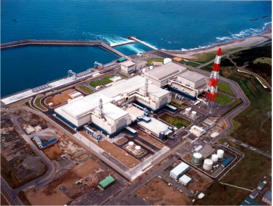
ABWR reactor at Kashiwazaki-Kariwa Nuclear Power Station, Japan
