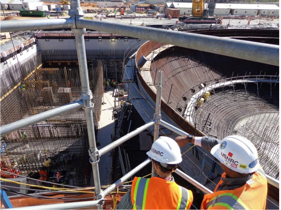
AP1000 reactor construction at Vogtle Electric Generating Plant, USA
